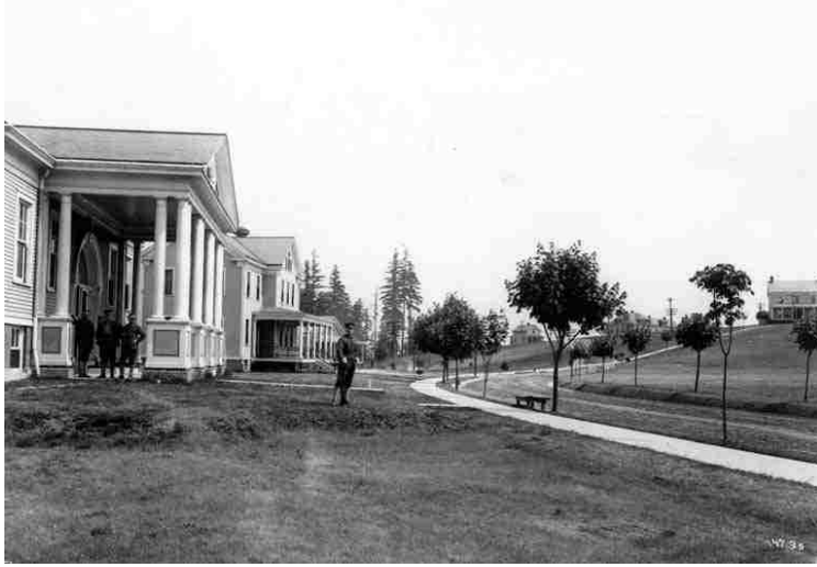
Figure 19. Parade Ground with Gymnasium, Band barracks, Administration Building (1909)
